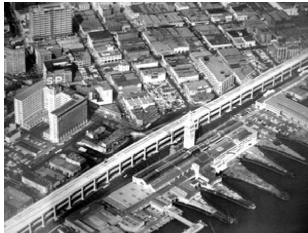
The Embarcadero Freeway, circa 1960, as it once existed along San Francisco's waterfront.
